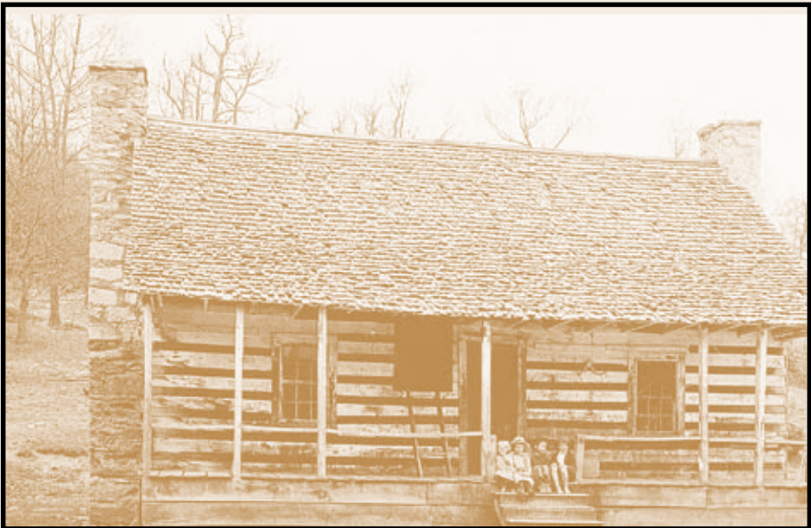
Children perch on the King house steps, which became home to Dr. Schenck's head rangers. Note the ladder and "scuttle hole" replaced by steps in the early 1900's.
